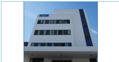
IBS INC. Japan head office & factory, Osaka, Japan
